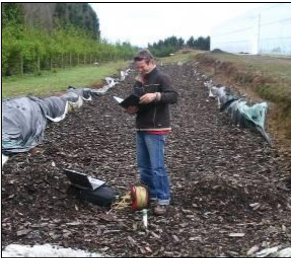
Above - large denitrification bed for treating discharge from a hydroponic glasshouse. 140 m long by 6 m wide and 2 m deep.
