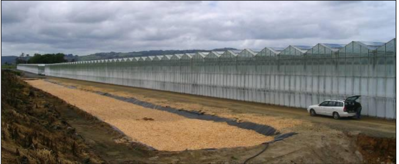
Above - large denitrification bed for treating discharge from a hydroponic glasshouse. 140 m long by 6 m wide and 2 m deep.
